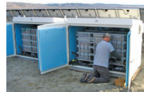
Large battery enclosure for MAPPS solar powered air monitoring system.
