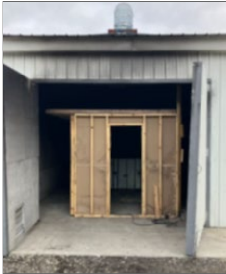
Figure 4: Photo 5 from Test Report Displaying Room Used for Testing
