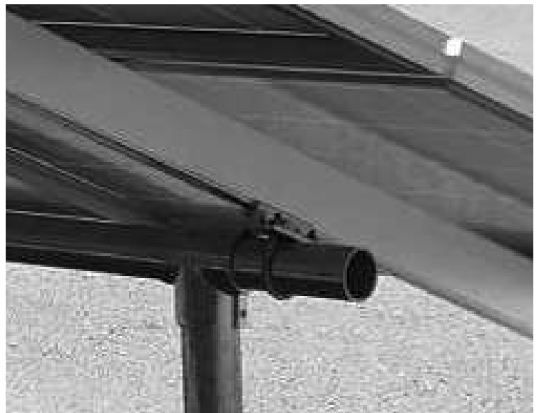
Attach Pipe Mount to Rail
